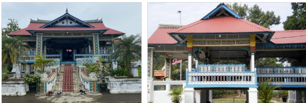
Fig. 2. Front façade (left), and part of side elevations of Melaka Malay traditional house (right)
