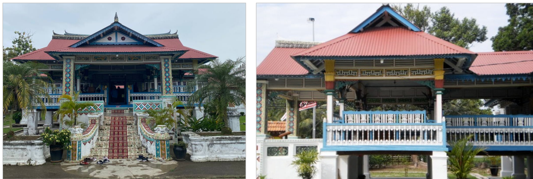
Fig. 2. Front façade (left), and part of side elevations of Melaka Malay traditional house (right)
