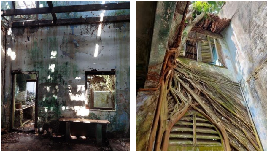
Fig. 4. The condition inside one (1) of the many Papan's lines of shophouses (left) and Pokok Banyan Berakar di Dinding, one (1) of the shophouses in Papan that has been grown by the root of a Banyan tree (right).
