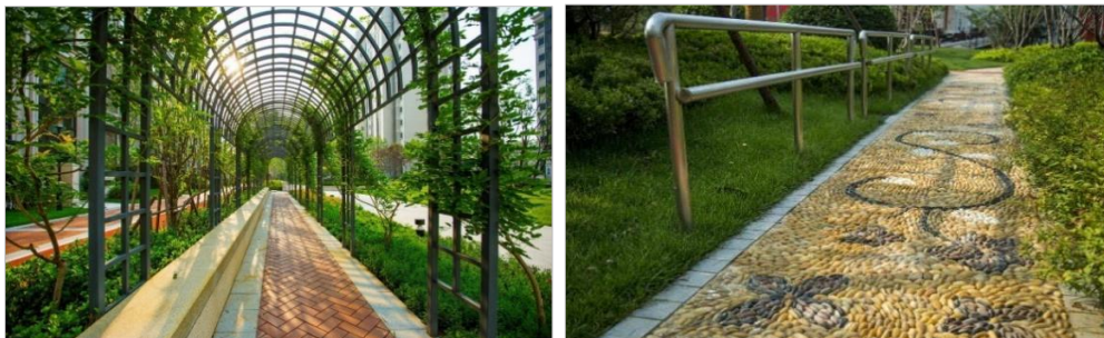
Fig. 6. Characteristic of suitable pavement design with rough surface of materials for elderly in Taikang Home, Yanyuan, China
