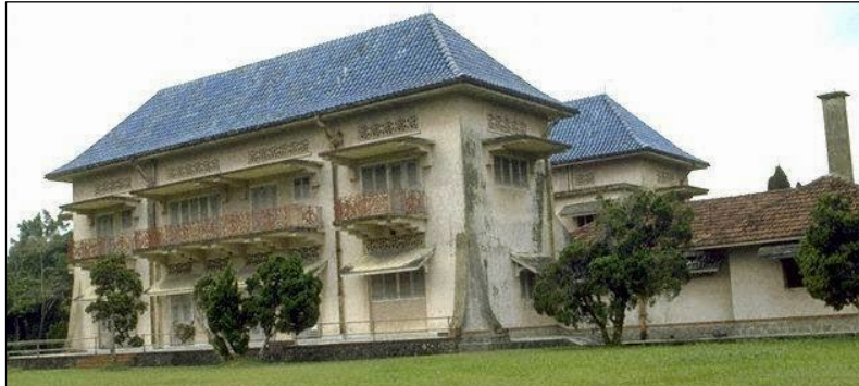
Fig. 13. The Building Façade of Istana Woodneuk, Singapore.
