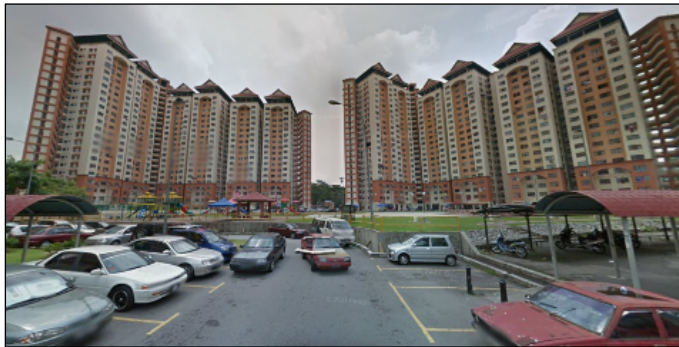
Fig. 10. Before construction of podium parking
