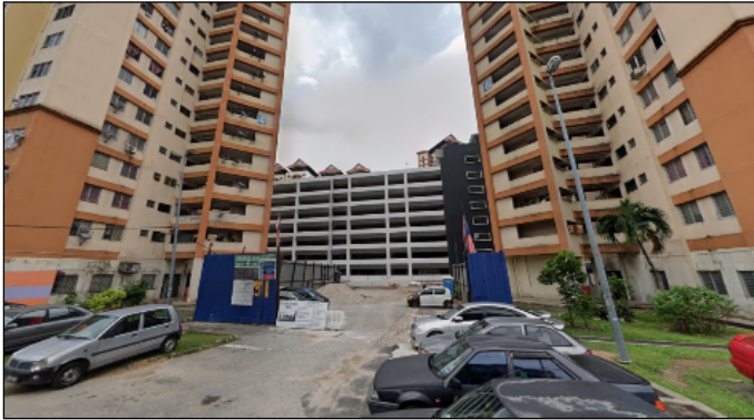
Fig. 11. After construction of podium parking
