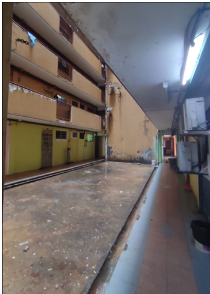
Fig. 2. Flat Internal Courtyard
