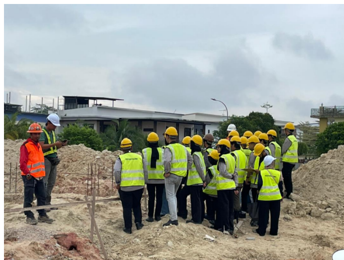
Fig. 3 Students observing the Excavation work.
