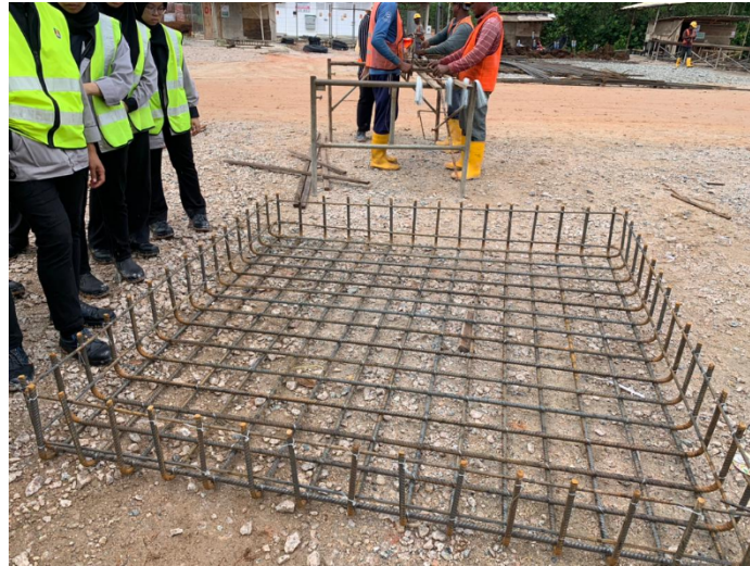
Fig.2 Students observing the process of reinforcement steel on site.
