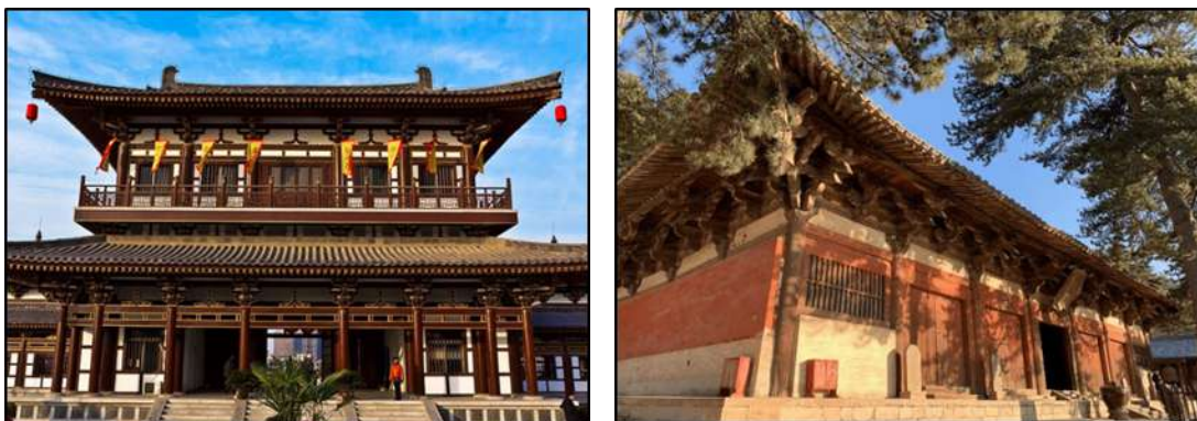
Figure 4. Tang Dynasty Architecture Qinglong Palace (left), and The Great Hall of the Buddha's Light Temple (right) (Source: Cai, 2011)
