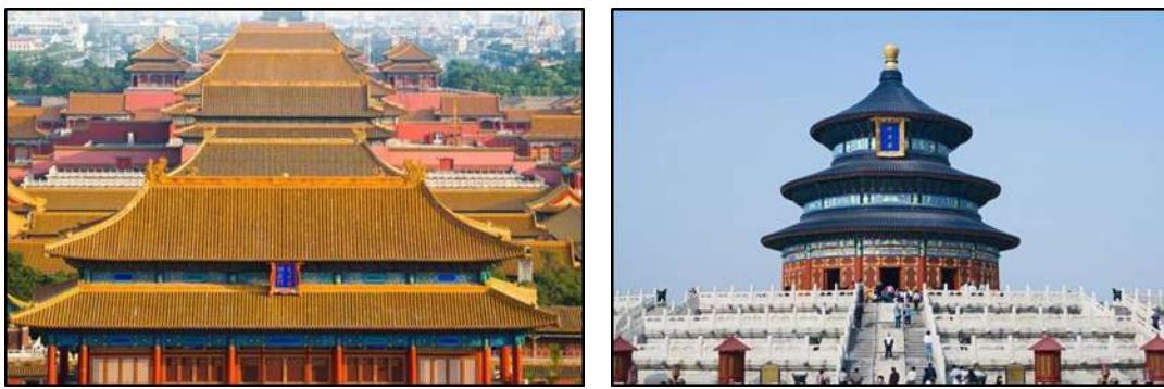
Figure 8. Yuan Dynasty Architecture Forbidden City (Qing) (left) and Temple of Heaven (Qing) (right)
