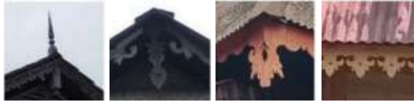
Figure 1. The roof decorative architectural components of RLBP (Source: Author' collection)
