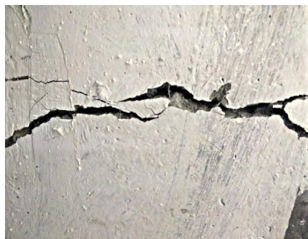
Figure 10: Crack Pattern of Failed Three-Ribbed Slab (source by author)
