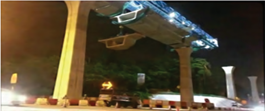
Figure 10: Gantry launcher used to lift the precast segments on-site (Respondent B)
