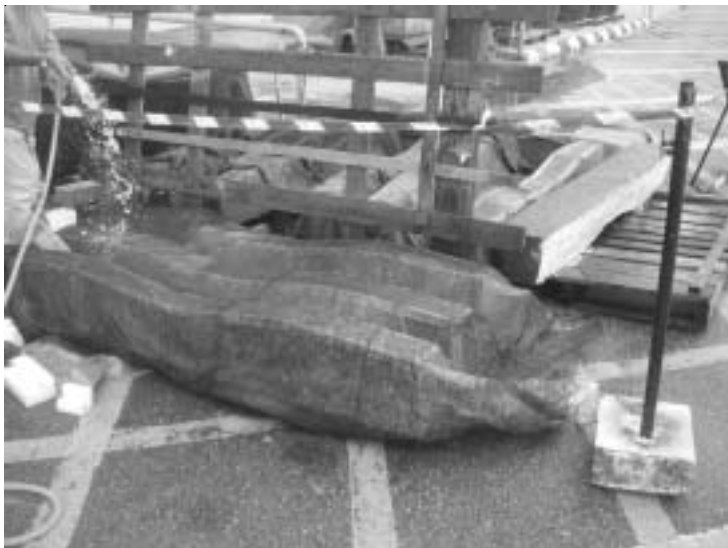
Plate 3: Curing of Sleepers
