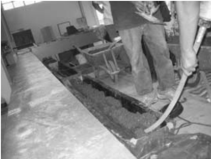
Plate 2: Concrete Placement in Moulds
