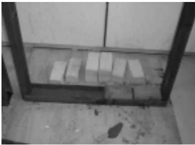
Photo 1: U shaped steel frame
